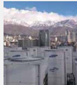
Location: Iran (Tehran) Project: Commercial Centre of Elahiye
