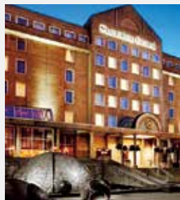
Location: UK (Edinburgh) Project: Sheraton Hotel
