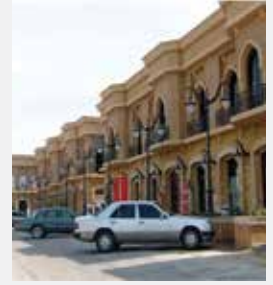
Location: Saudi Arabia Project: Medical Clinic
