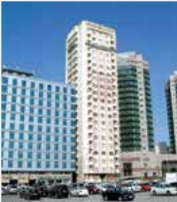
Location: Qatar Project: Office Building
