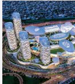
Location: Turkey (Istanbul) Project: Mall of Istanbul
