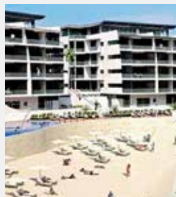
Location: Kenya (Mombasa) Project: English Point Marina
