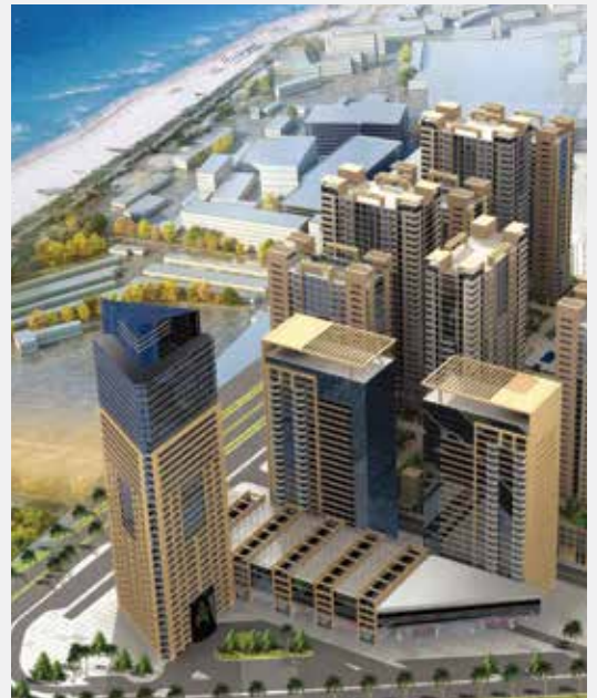
Location: UAE Project: Residential Building
